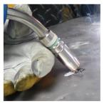
Ideal for Aluminum repair. Photo of 0.8mm thick Aluminum weld I-CAR test.
